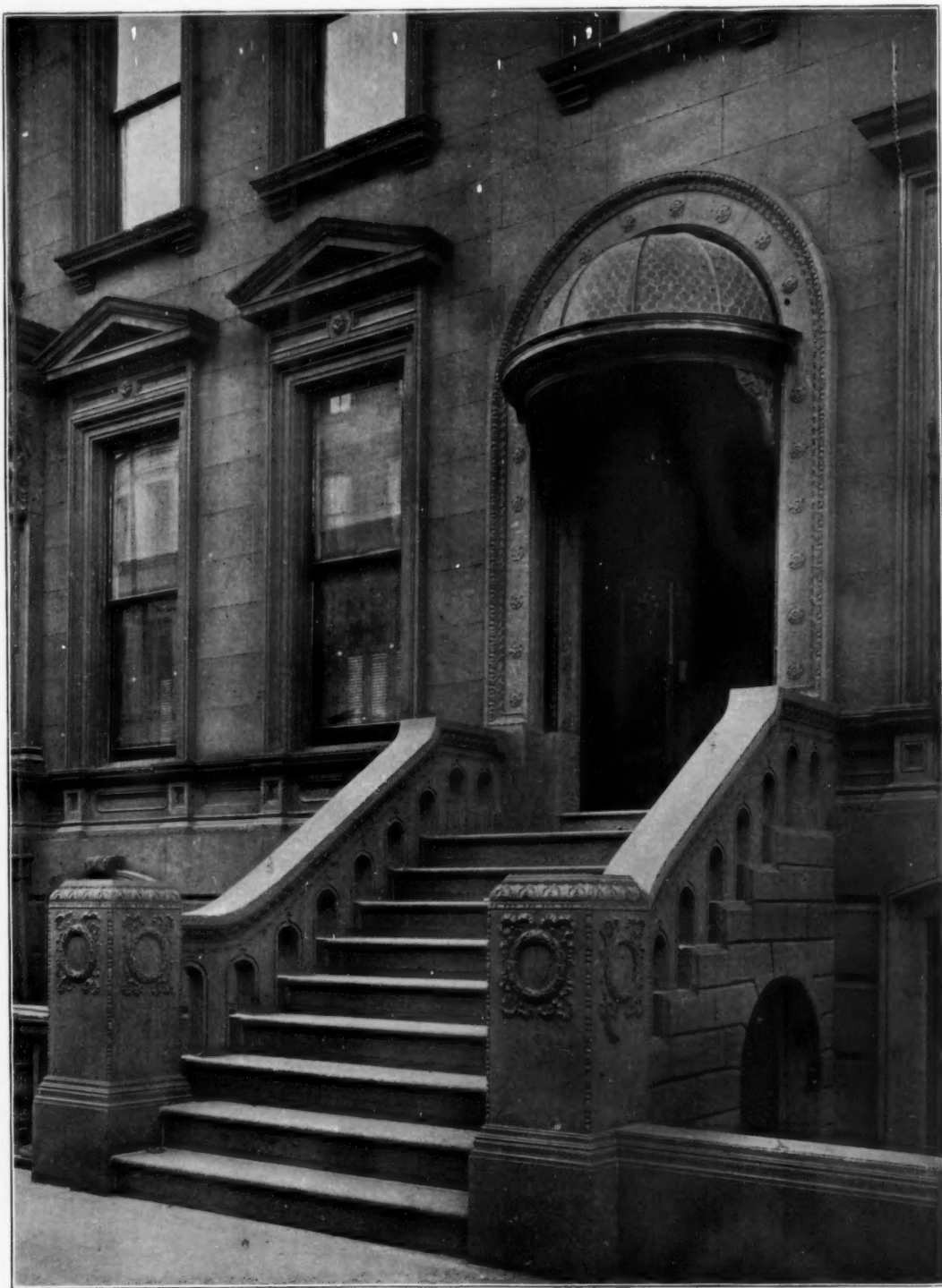
FRONT STEPS.—No. 6 EAST 38TH STREET, NEW YORK, N. Y.
