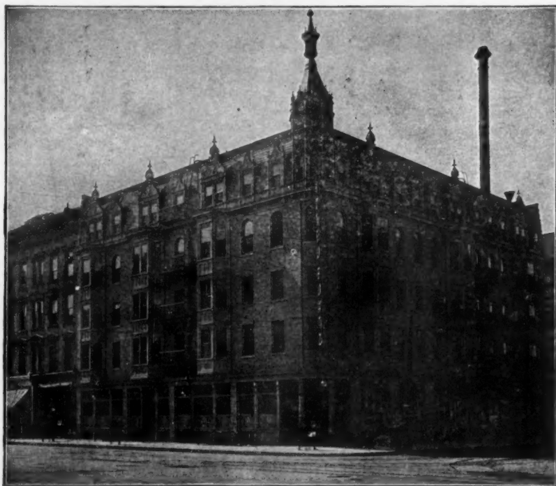
BLATZ HOTEL, MILWAUKEE, WIS. OTTO STRACK, ARCHITECT.
