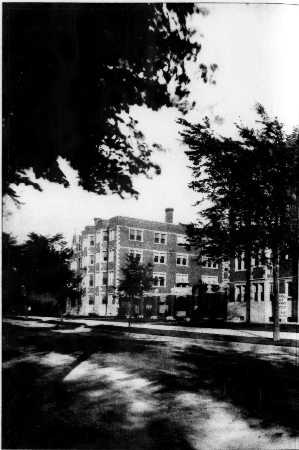
RICHMOND COURT APARTMENT CRAM, GOODHUE & FERRIS
