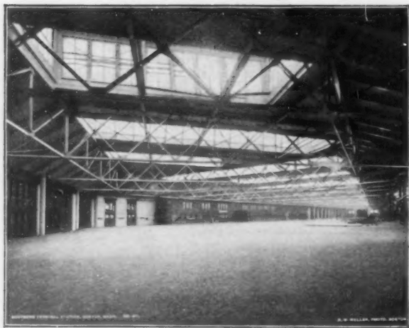
"The Midway" between the Head-house and the Train-shed.
