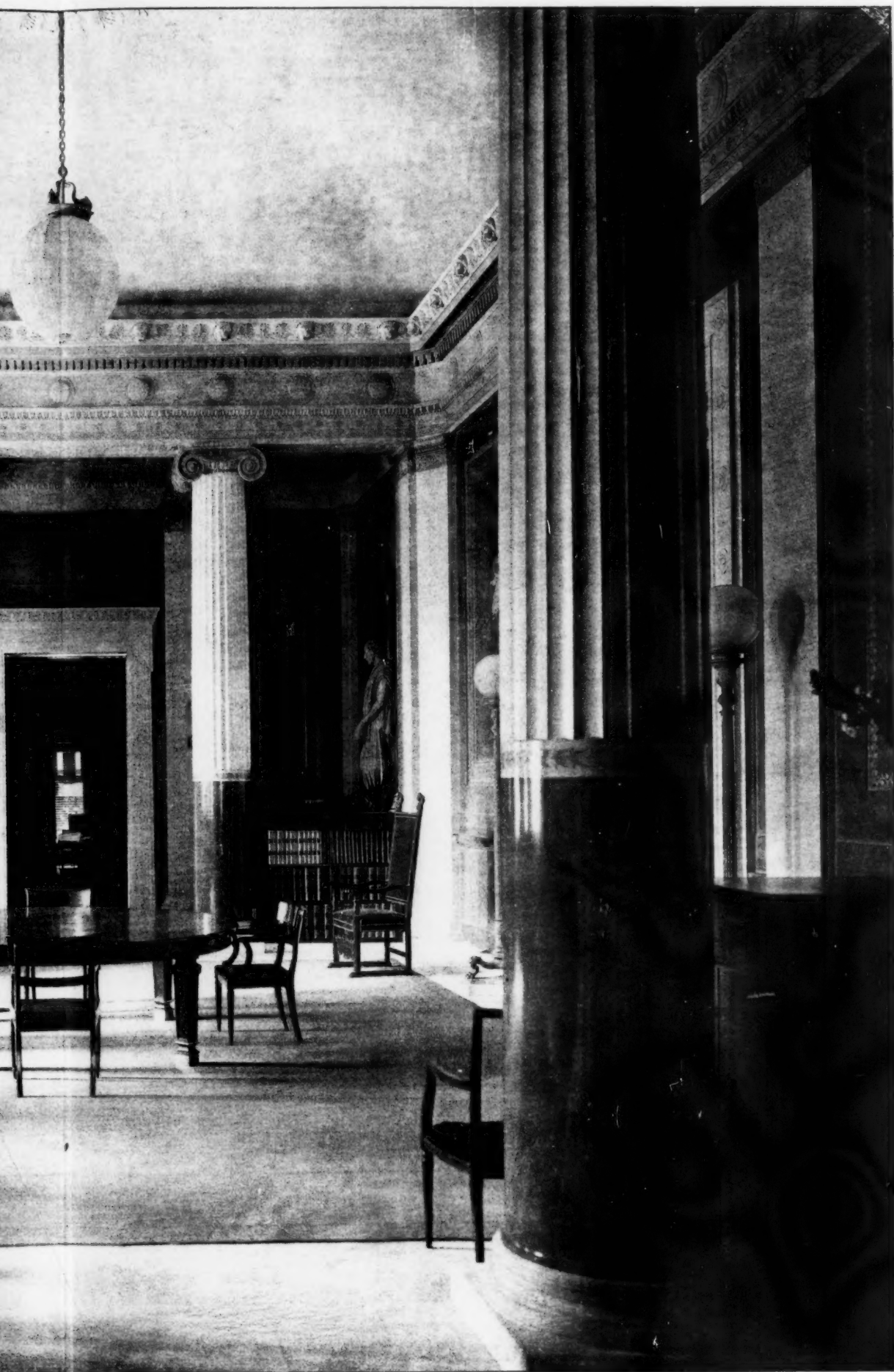
BRARY: UNIVERSITY CLUB, NEW YORK, N. Y. HEAD & WHITE ARCHITECTS.
