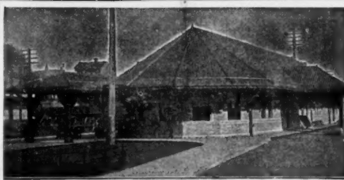
N. Y. Central R.R. Depot at Amsterdam, N. Y., Roofed with Merchant's Copper "Spanish" Tiles.
