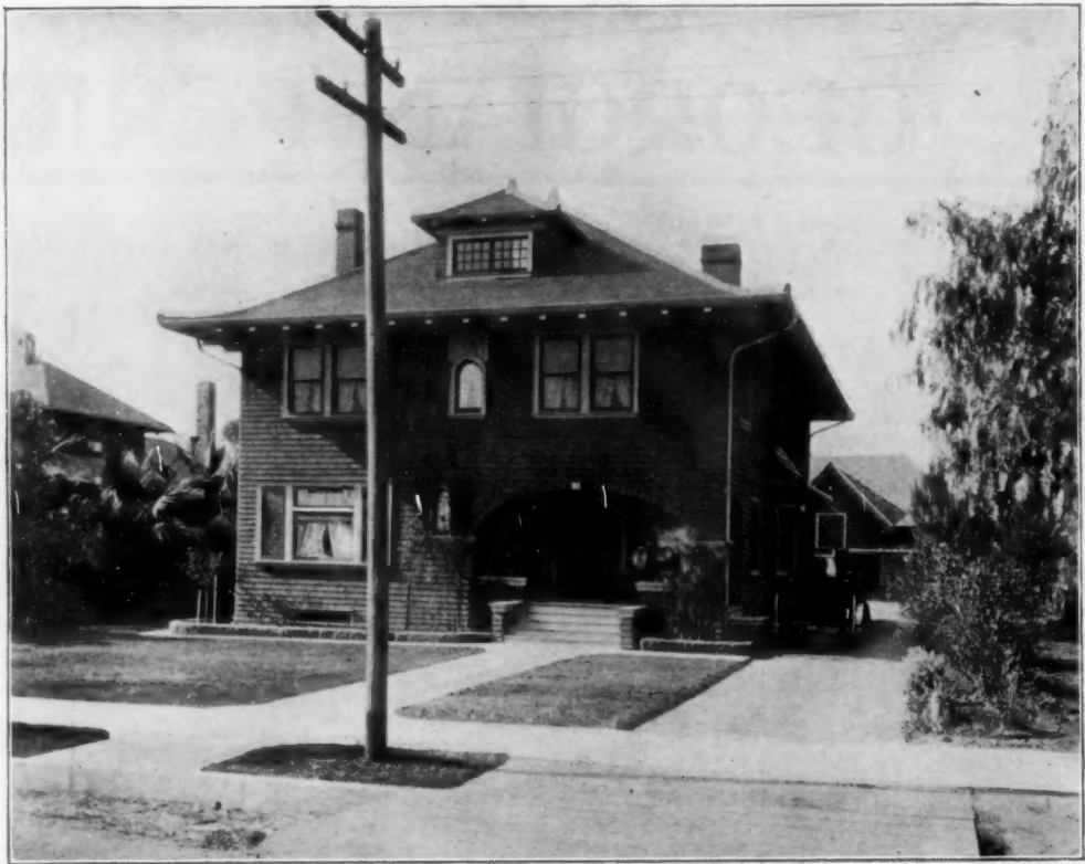
HOUSE OF W. H. ALLEN, ESQ., PASADENA, CAL. BLICK & MOORE, ARCHITECTS.
