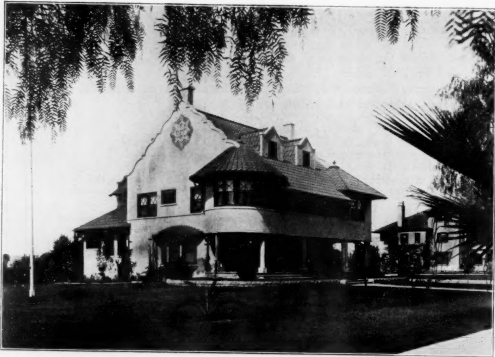
HOUSE OF J. H. ADAMS, ESQ., PASADENA, CAL. ADAMS, PHILLIPS & CO., ARCHITECTS.
