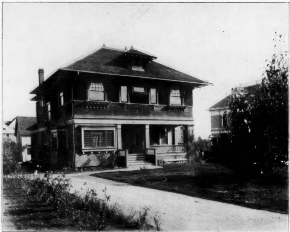
HOUSE OF MR. DURRELL, PASADENA, CAL. BLICK & MOORE, ARCHITECTS.
