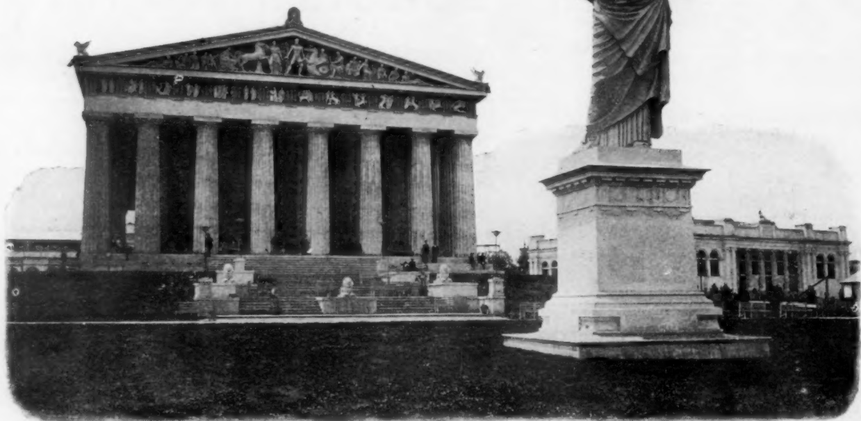
Tennessee Centennial Buildings, Nashville, Tenn. Art Building: W. C. Smith, Architect.
