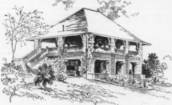
Shelter at Charlestown Heights.
