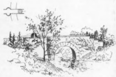
The Riverway: A Foot-bridge near Bellevue St.
