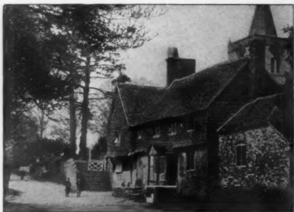
Old House at Willey, near Guilford, Eng.
