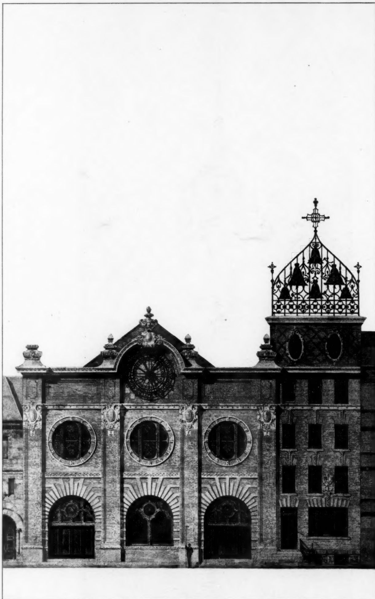
NEW FRONT: CENTRAL METHODIST EPISCOPAL CHURCH, NEW YORK CITY.
