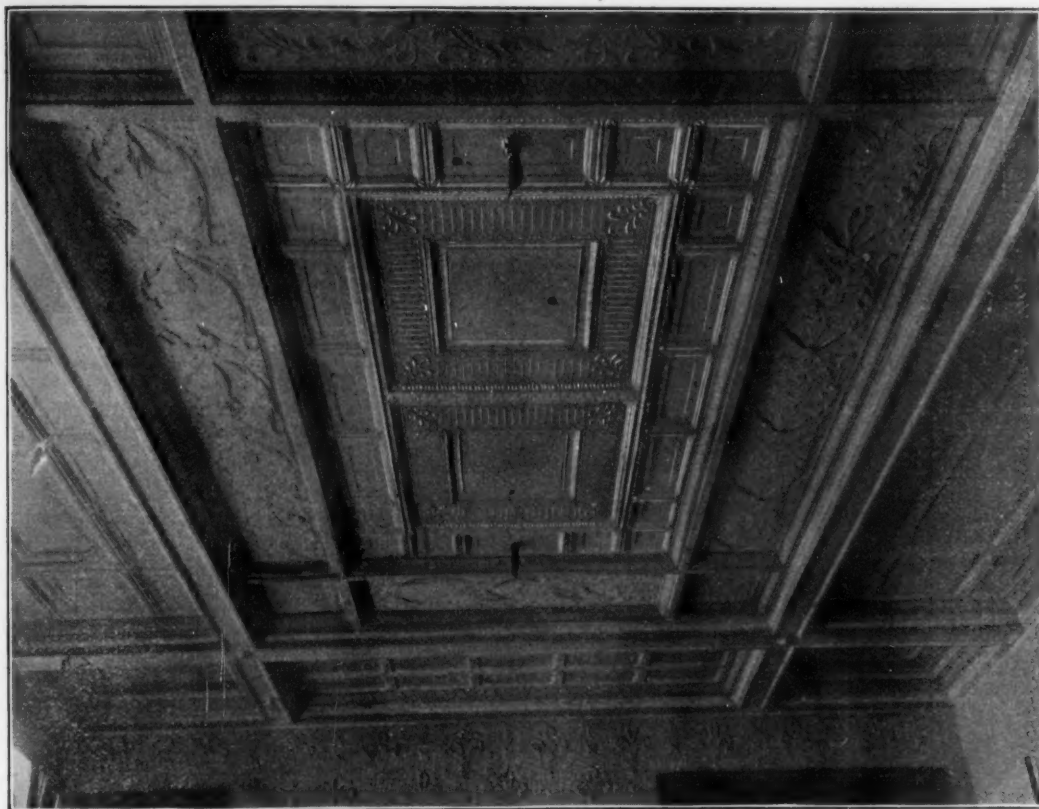
Showing Nos. 22 and 25½ Panels and No. 1 Border with No. 26 special Moulding and encased beams.
