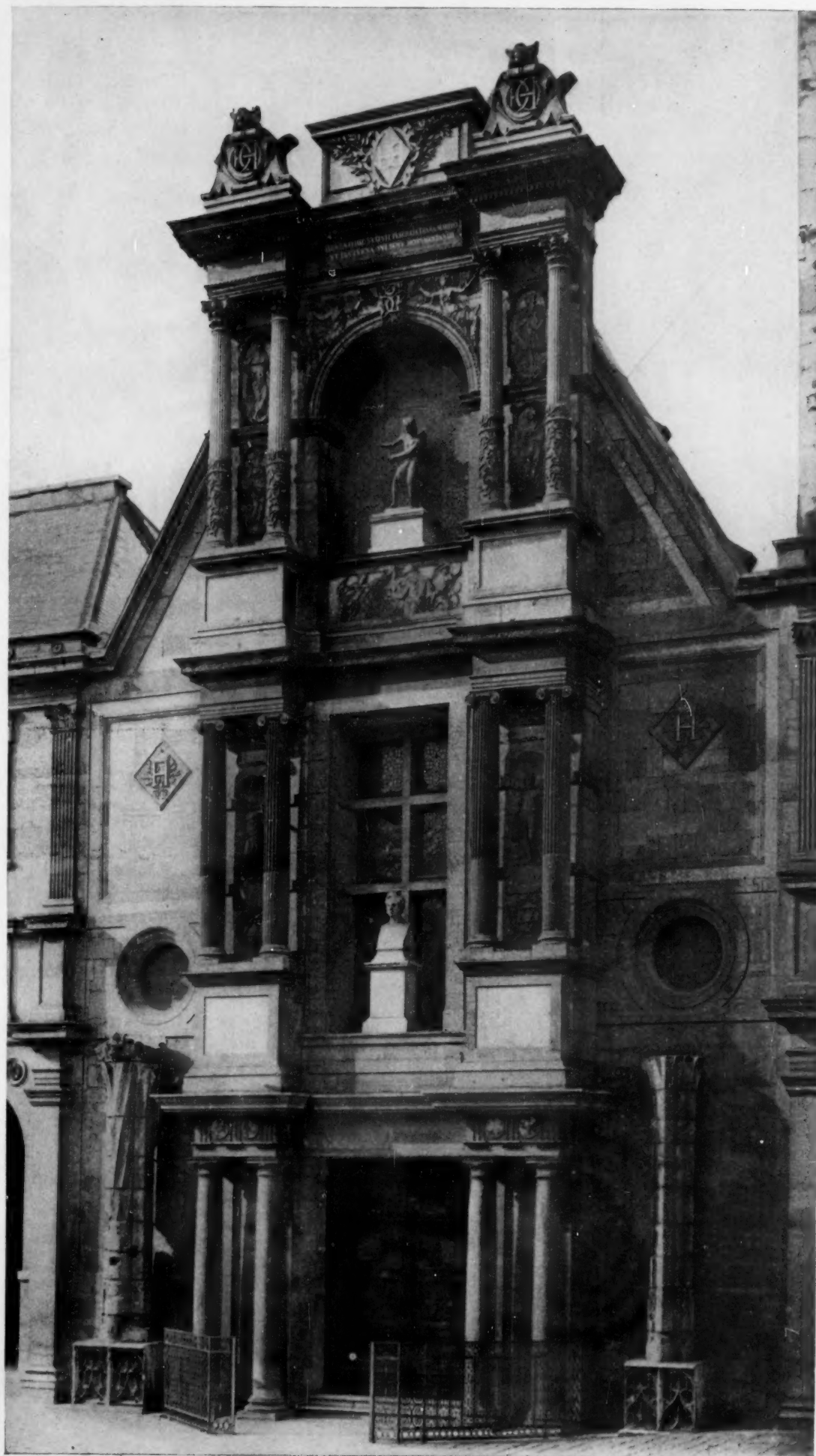
FACADE OF THE CHAPEL OF THE CHÂTEAU D'ANET.
