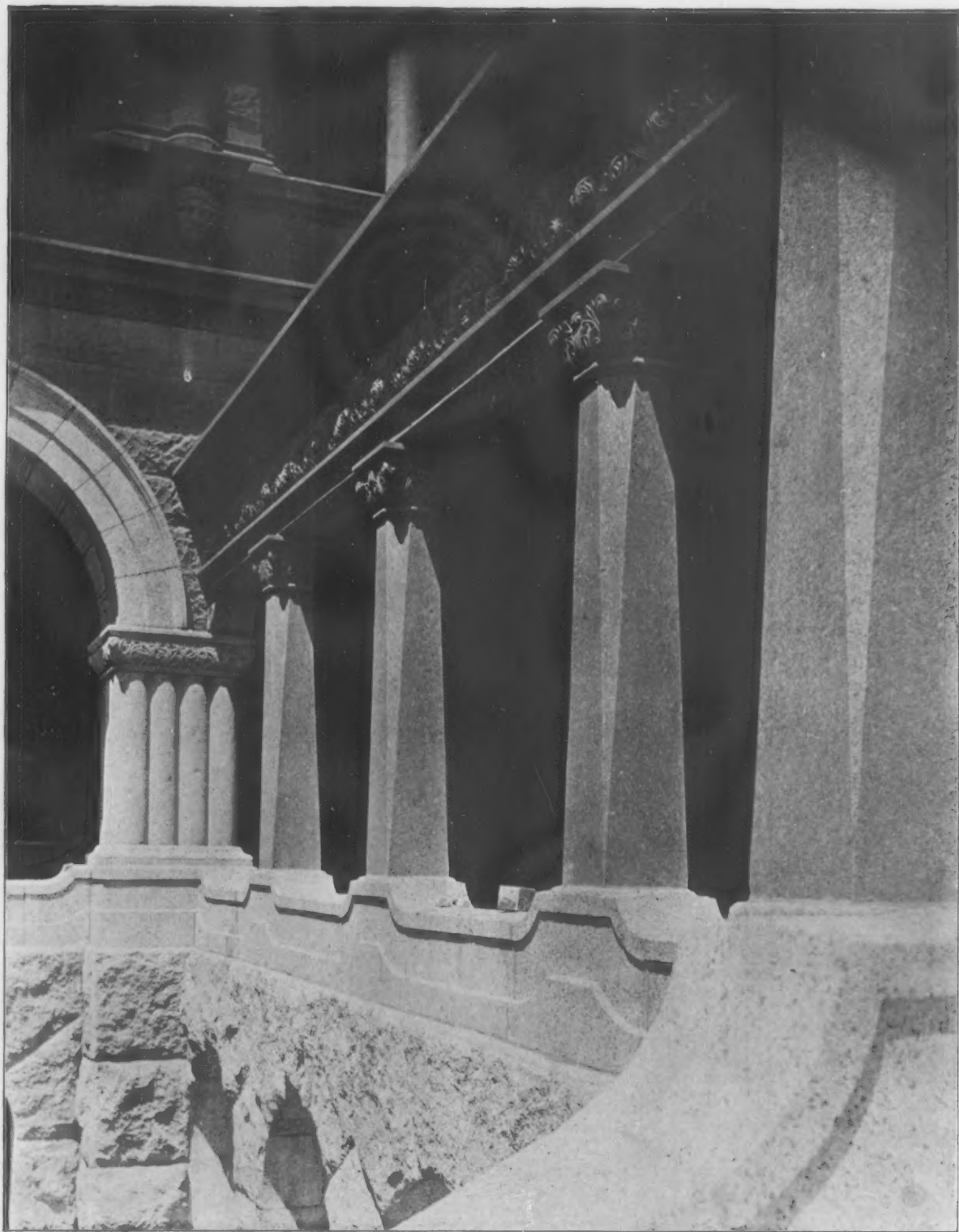
DETAIL OF BEXAR COUNTY COURT HOUSE, SAN ANTONIO, TEX.
