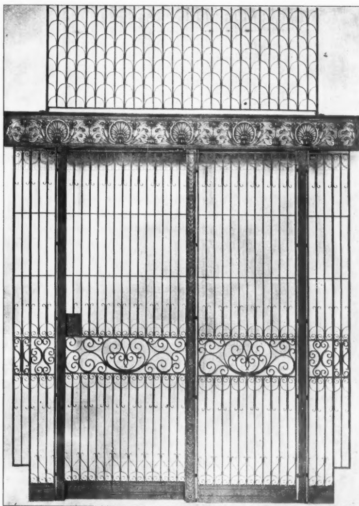
FIRST-STORY ELEVATOR SCREEN.
