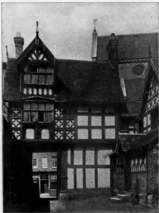
The Council-House, Shrewsbury: looking out.
