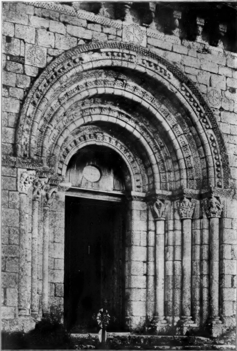
DOORS AND DOORWAYS, No. 5:—WEST DOOR OF THE CHURCH OF ST. MICHAEL, LESCURE, TARN-ET-GARONNE, FRANCE.
