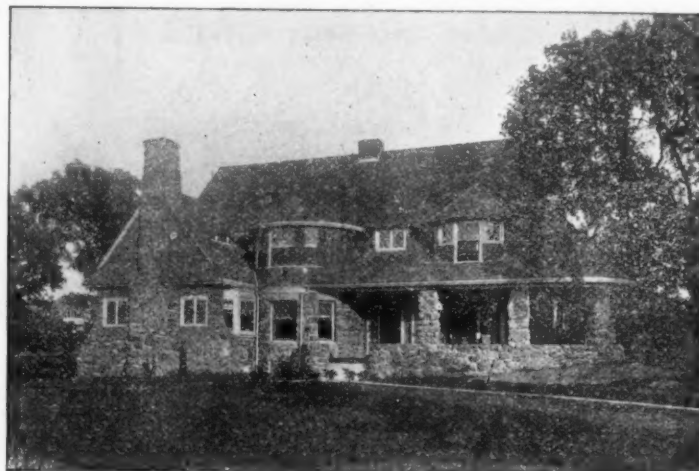
CHAPMAN, FRAZER &amp; BLINN, ARCHITECTS, BOSTON.
