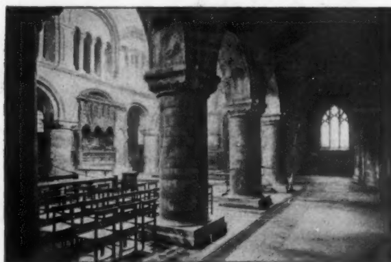
View from South Ambulatory, looking East.
