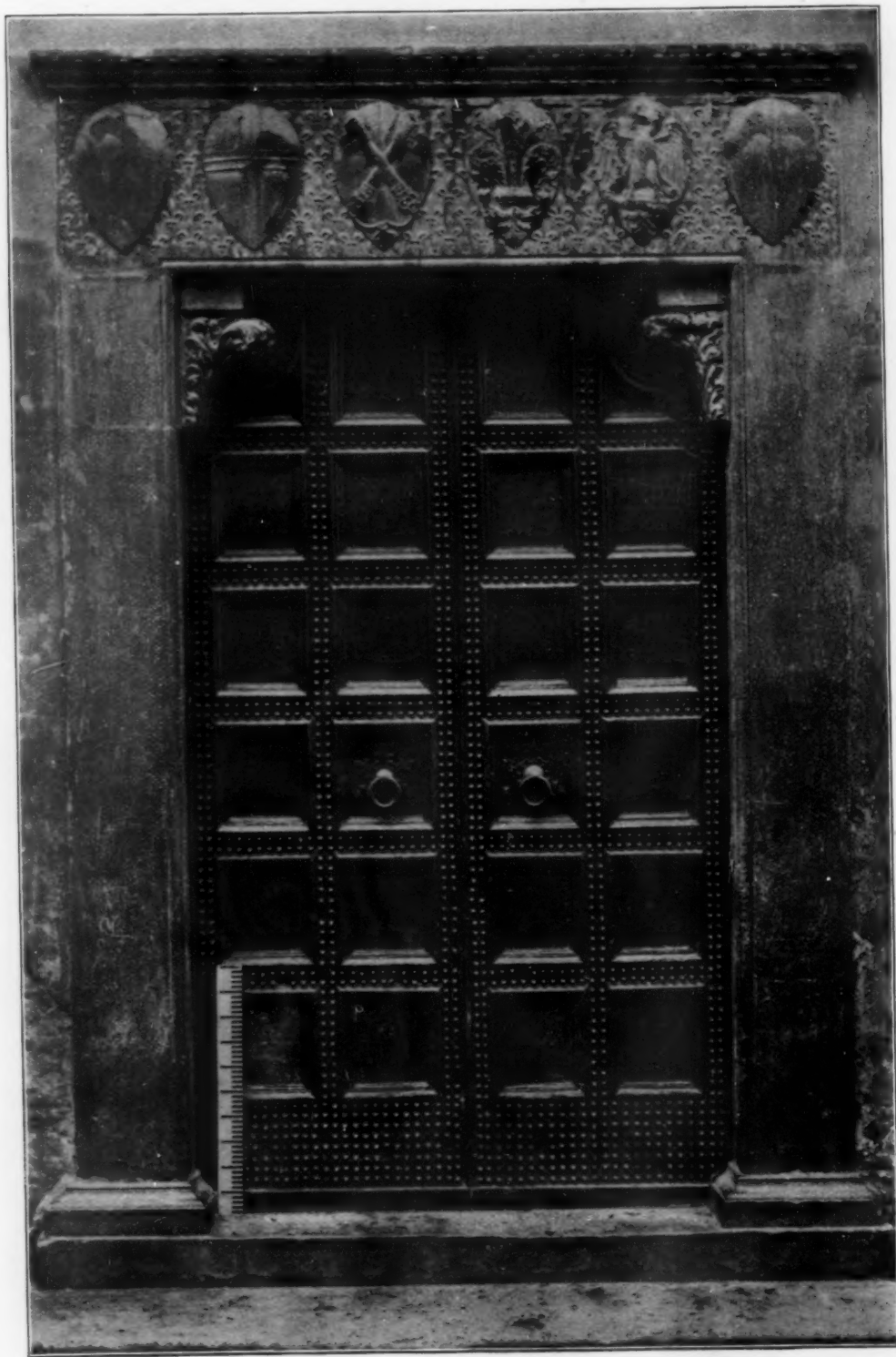
DOORS AND DOORWAYS, No. 1:—DOOR OF A HOUSE ON THE PIAZZA S. ANDREA, IN THE MERCATO VECCHIO, FLORENCE, ITALY.
