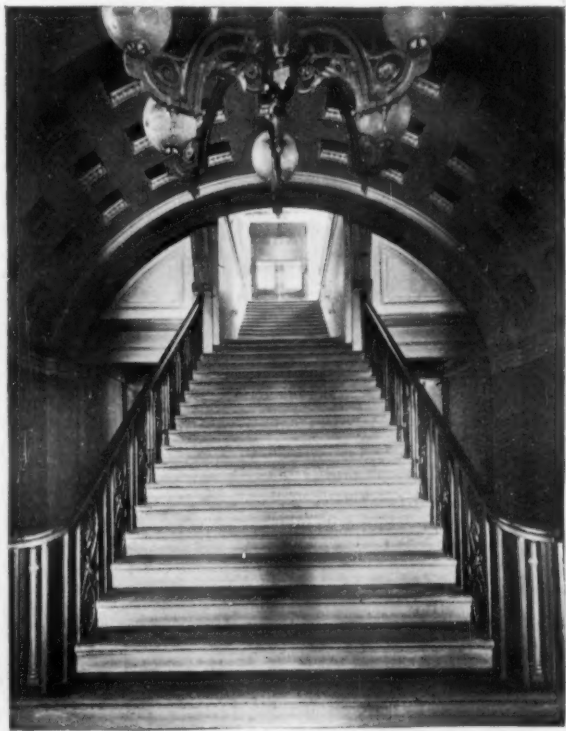
Fig. 69. Principal Stairway from Basement.
