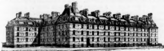
Fig. 13. Gatliff Buildings, London, Eng.
