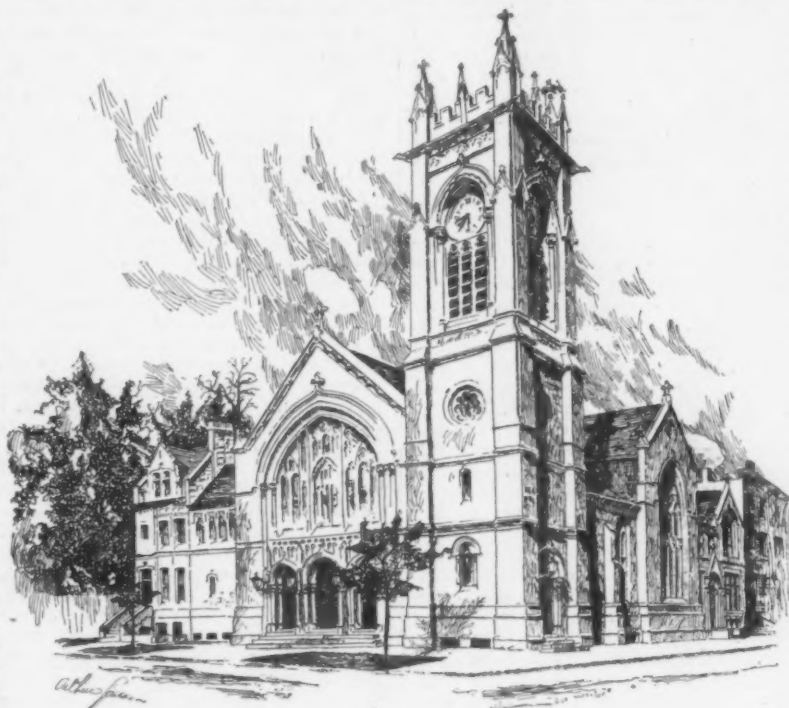
Fourth Presbyterian Church, N. Y. Messrs. Heins &amp; LaFarge, Architects.
