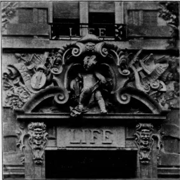
Door-head, Life Building, New York, N. Y. Carrere &amp; Hastings, Architects.
