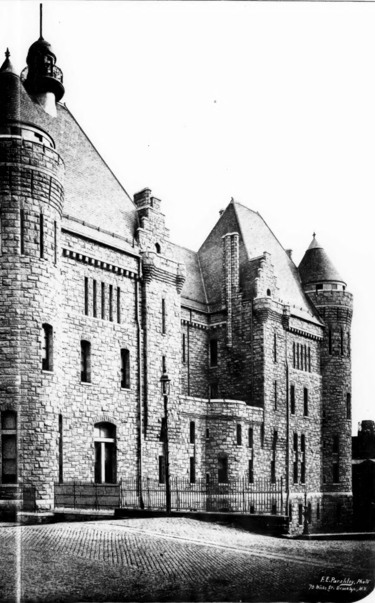
N. Y., PARK AVENUE AND THIRTY-FOURTH STREET, NEW YORK, N. Y.
