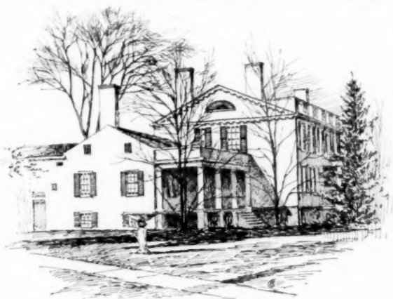
House at Canandaigua, N. Y.
