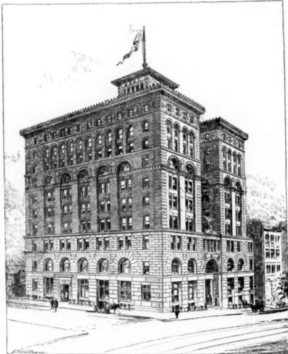
New York Life Insurance Building, Omaha, Neb.: Private Architect. Total cost, $833,399; Cost per cubic foot, 39 cents; Time of Construction, 24 months.
