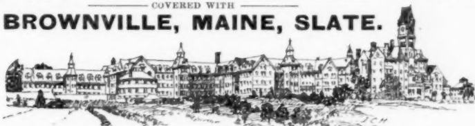
Brownville Maine Slate Co., Worcester, Mass.
