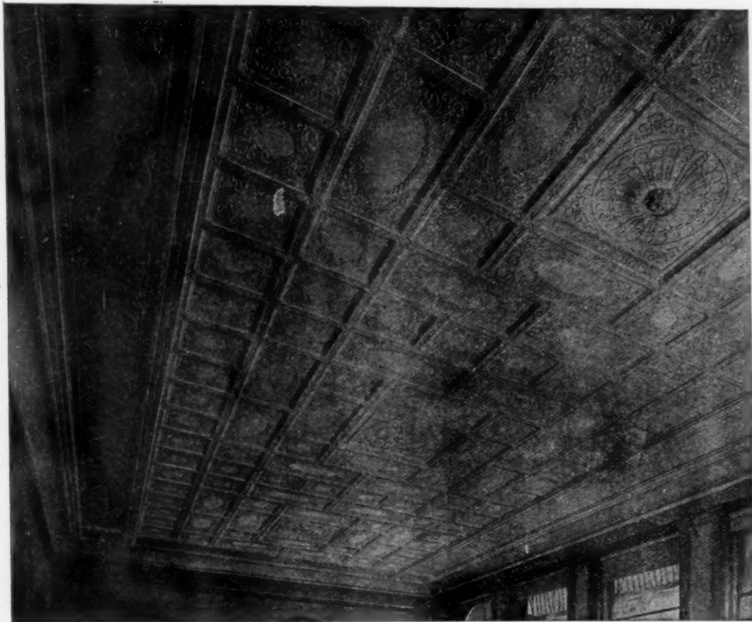
Steel Ceiling in the First National Bank, Paterson, N. J. Manufactured by H. S. Northrop.
