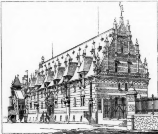
Fig. 36. Custom-House, at the Railway Station of Tournai.
