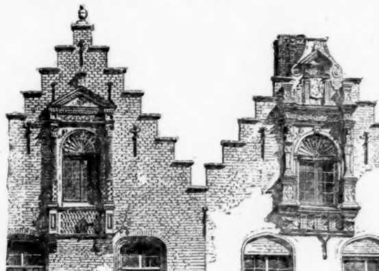
Fig. 26. Windows at Furnes.
