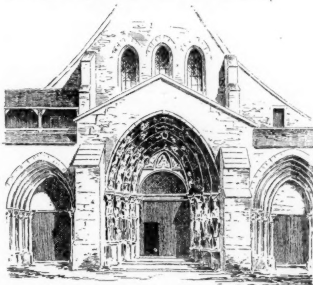
Fig. 14. Portal of Saint-Ayoul, Provins.
