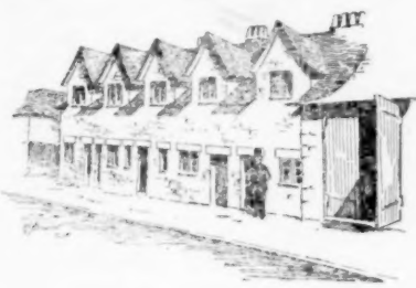
Workmen's Cottages, Ross.
