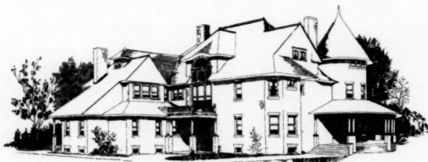
View from the Northwest
