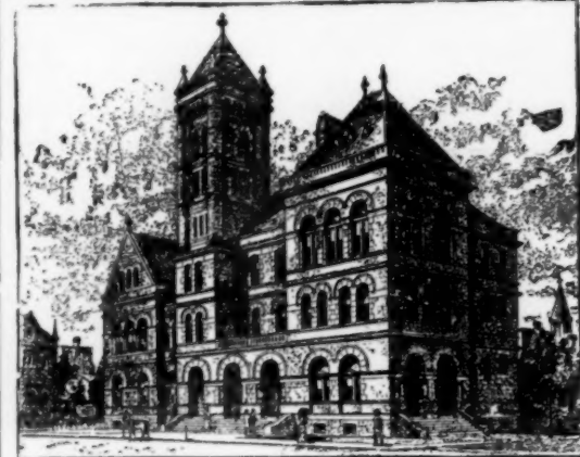
U. S. Court House and Post Office, at Williamsport, Pa., Plastered with King's Windsor Cement.
