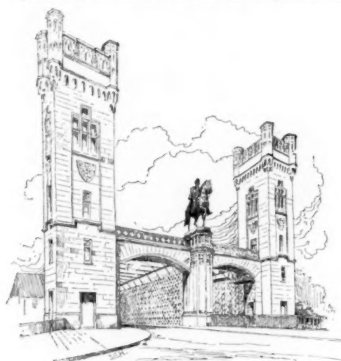
Entrance to the Iron Bridge from the Cologne Side.
