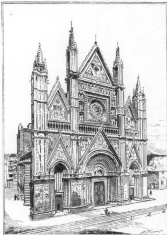
Fig. 14. Façade of the Cathedral of Orvieto.
