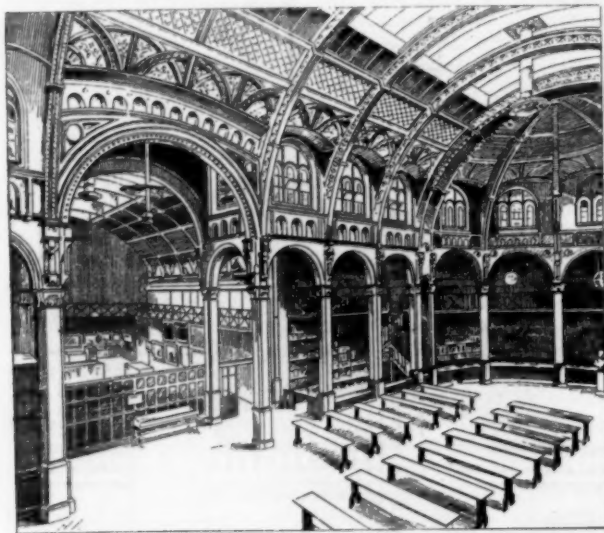
Fig. 26. Interior View of the Library at Birmingham.
