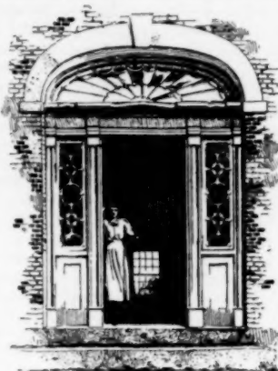
Front Entrance to "the Brick."
