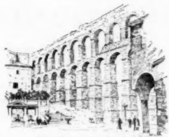
Aqueduct at Segovia.
