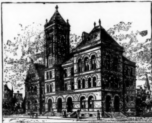
U. S. Court House and Post Office, at Williamsport, Pa., Plastered with King's Windsor Cement.
