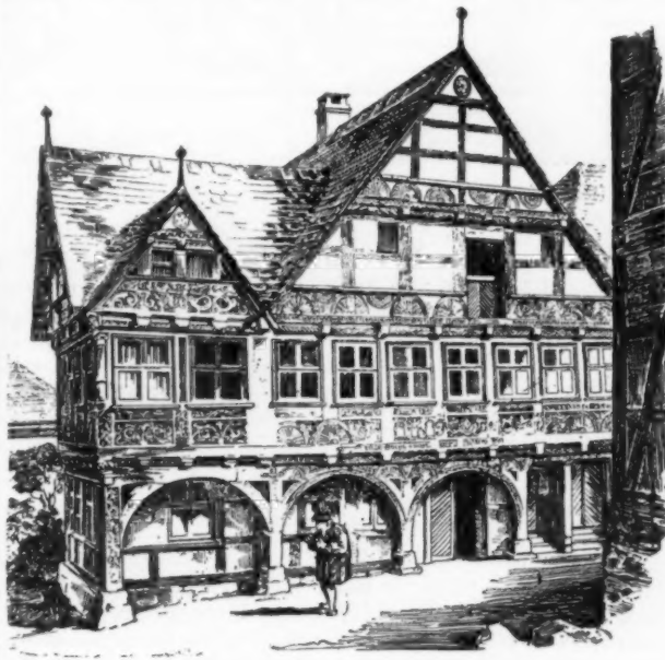
Fig. 47. Town-hall at Schwalenberg.
