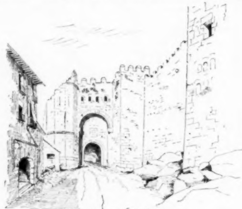
THE WALLS - SEGOVIA
