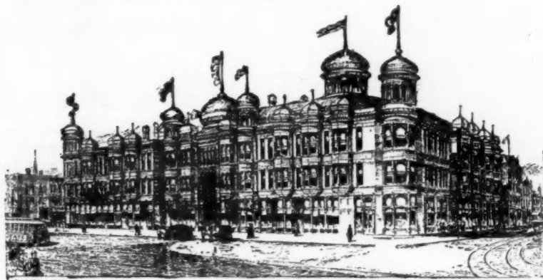
Covered with the Genuine Taylor "OLD STYLE" Brand of Roofing Tin.
