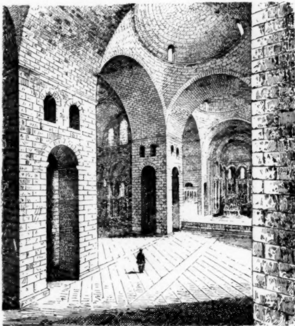
Fig. 7. Interior of St. Front, at Périgueux (10th Century).
