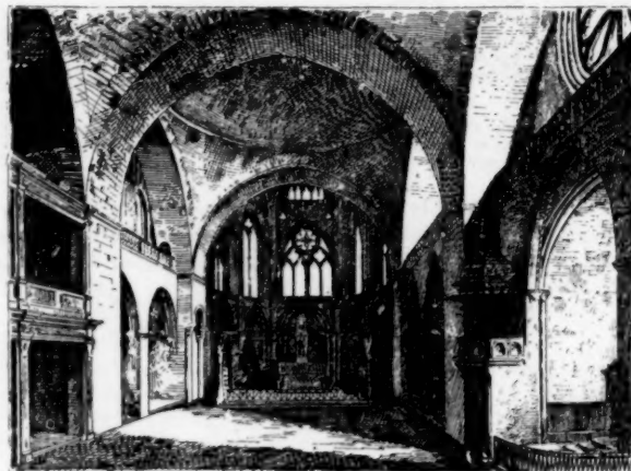
Fig. 10. Interior of the Church of Cahors. After M. de Verneilh.
