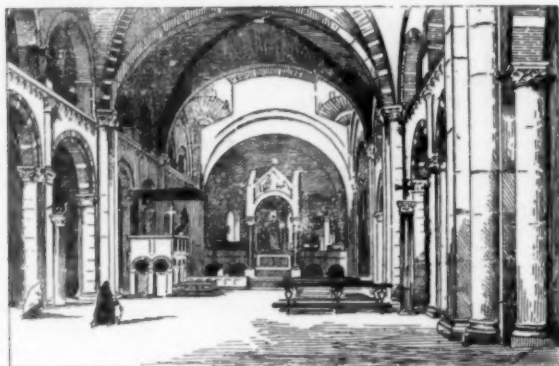
Fig. 5. Interior of S. Ambrogio, at Milan.
