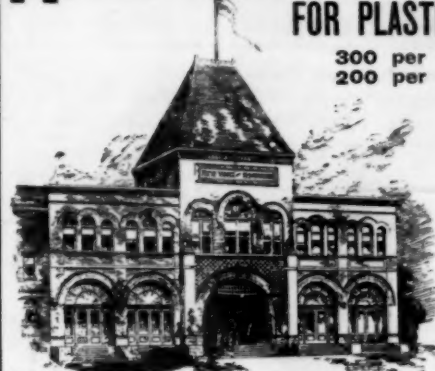
Station of the N. Y. City and Northern B. R., Yonkers, N. Y., Plastered with King's Windsor Cement.
