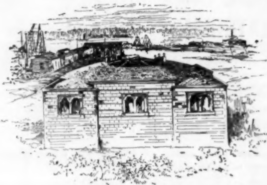
[Dome 40 feet in Span and 2 inches thick.]
