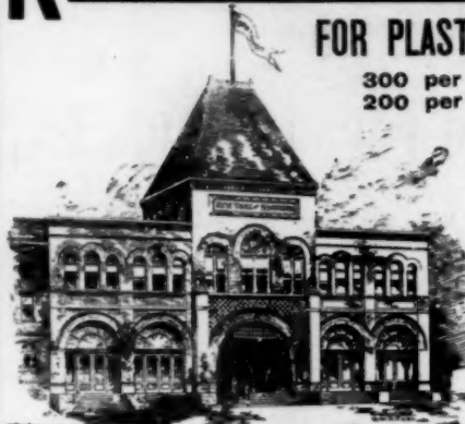
Station of the N. Y. City and Northern R. R., Yonkers, N. Y., Plastered with King's Windsor Cement.
