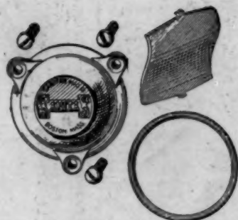
Sanitas Trap - Cup, Partition, and Washer.
