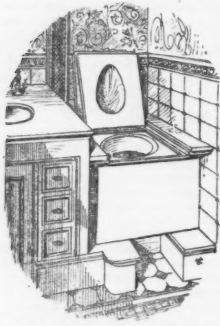
Fig. 34.—Combined Urinal and Water-Closet.
