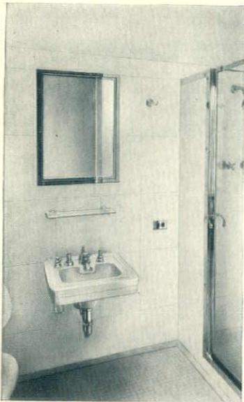
(Left) A Private Toilet and Bath—Crane NORWICH vitreous china lavatories with liquid soap faucets, ice water faucets, SECURO lever-action wastes and METRO slow-closing supply valves. Crane shower fixtures. Crane PURUS JR. closets with ALPHA flush valves.
