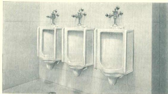
Men's Public Toilet No. 1—Crane RIO vitreous china wall urinals with foot-operated ALPHA flush valves, EXPEDIO wall closets with ALPHA flush valves.
