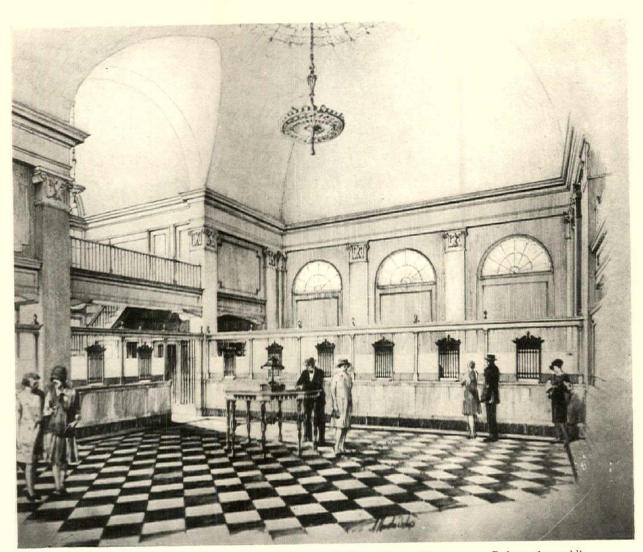
Above, the architect's preliminary perspective of the main banking room. Below, the public space of the main banking room as executed. The wall surfaces, pilasters, and vaulted ceiling are painted an old ivory, the ceiling being of a lighter shade than the walls. The floor is of Tennessee marble, the counter screen being of marble with a maple top screen and bronze wickets
