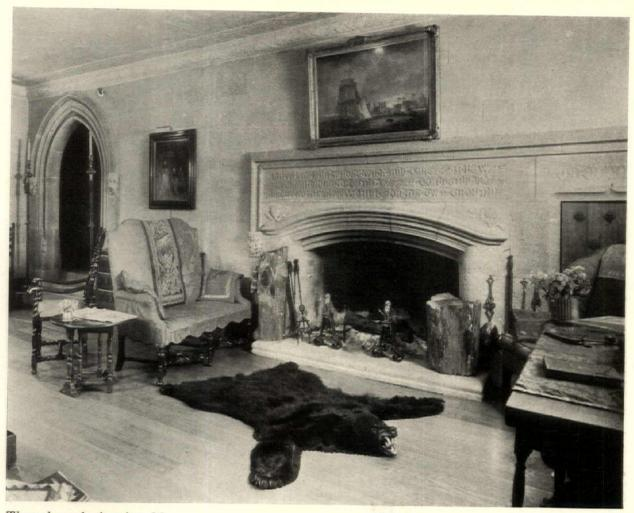
Throughout the interior, Mr. Hopkins has sought a feeling of masonry structure rather than the usual plaster veneer. These walls are of cinder block, painted a very light buff with a cold-water paint. The stone of the fireplace is all cast
