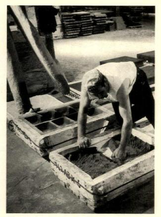
The pressing department. Here the plastic clay is pressed into the plaster moulds. The clay walls are usually about one inch thick with webs to give the necessary strength and stability
