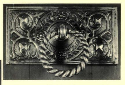
When it is an advantage to conceal the actual means by which the rim lock is secured to the door, the ingenious craftsman has a problem in which he revels. Often ornamented screw heads, or false screw heads, are resorted to, but here the raised leaf portions do the trick
