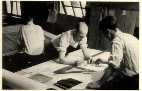
Making shop drawings of full-size details as derived from the architect's drawings. All full sizes, of course, are measured with a terra-cotta shrinkage scale—13 inches equal 1 foot
