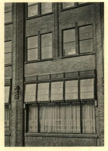
accompanying sketch (left) indicates the skilful manner in which this pier is laid. The intermediate piers and mullions carry the vertical enrichment across the façade, and prevent its being stranded on the widely spaced large piers. The color of the brick varies from pinkish red to yellow ochre. Below, a detail of the intermediate piers
