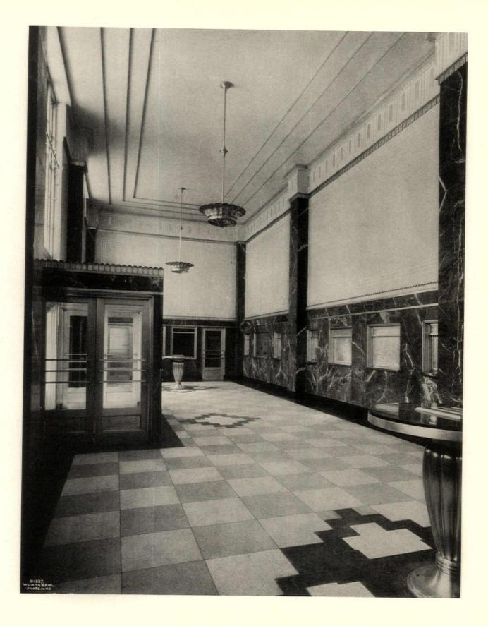
The public space is developed in a color scheme of several greens and aluminum. The floor is of terrazzo. Aluminum appears in doors, grilles, check desks, and lighting fixtures
