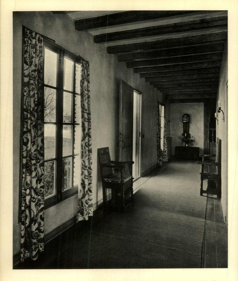
A view through the long hall looking towards the stairway. The ceiling beams are of roughly hewn oak, the floor of oak planks, and the plaster, hand worked with an integral brown coloring. To the hangings is entrusted the task of providing strong color
