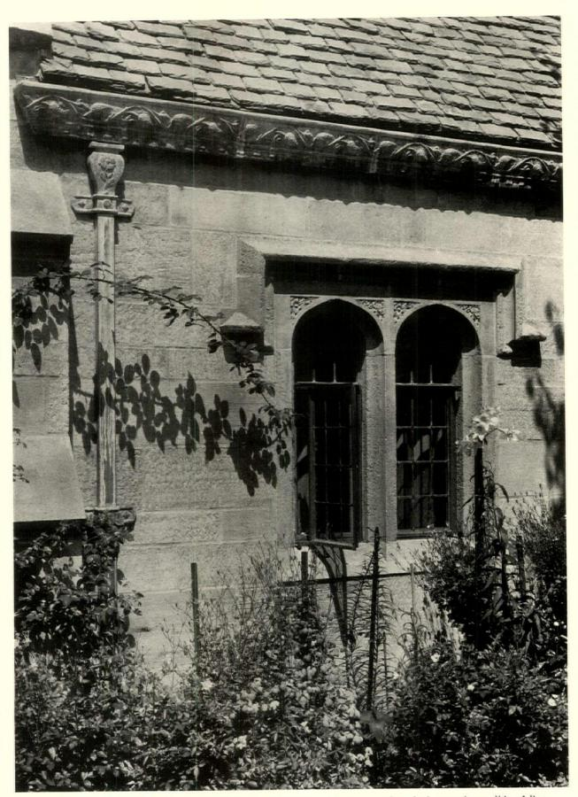
Mr. Hopkins has achieved a remarkable unity in his stone work, even though the exterior wall is of limestone, and the mullions and trim are of cast stone. The latter were made by a wax-mould method which avoids any suggestion of a moulded product. The gutter and downspouts are of lead-coated copper
