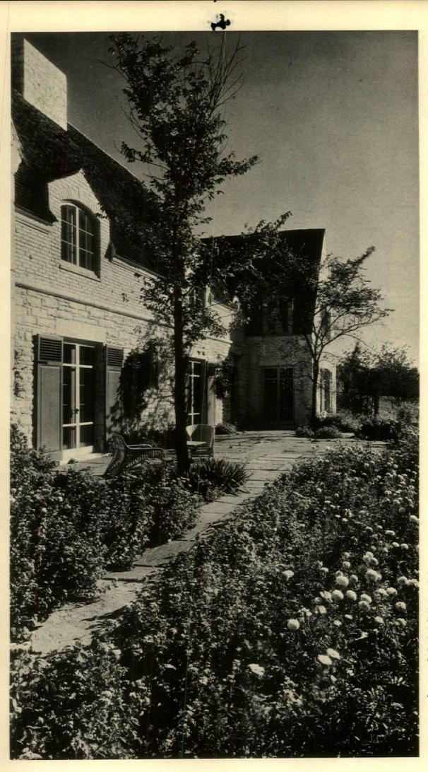
A local field stone is used for the first-story walls between the bays; this, the brickwork, and the cast concrete being covered with white wash in which there is a trace of yellow ochre. The terrace paving is of variegated flagstones
