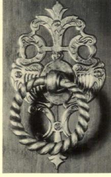
For certain periods of architecture or furniture it is sometimes advantageous to introduce the yellow color of brass, and while this material is usually thought of as being primarily suitable for casting, it also is excellent for hand tooling, as is evidenced by this rim lock
