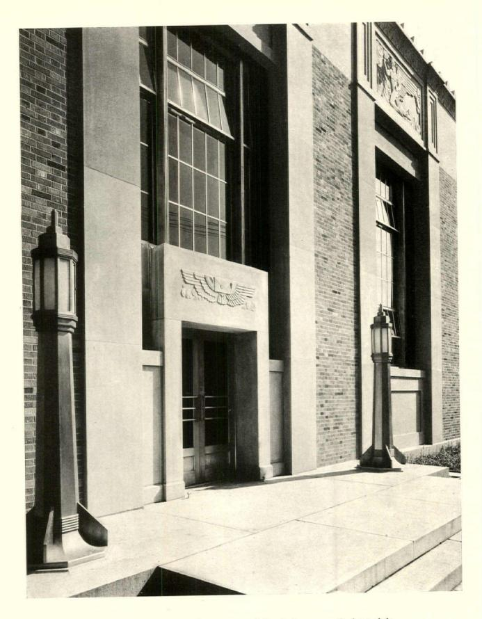
The metal work of the main entrance and the windows across the front of the building are of aluminum, as are also the lighting standards flanking the main entrance. The sculptured panels over the windows, and the abbreviated cornice, are of limestone
