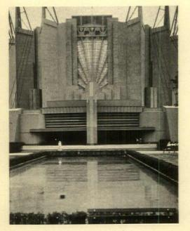
The "breathing dome" of the Travel and Transport Group; the dome is hung from steel posts guyed with steel cables. Edward H. Bennett, Hubert Burnham, John A. Holabird, architects
