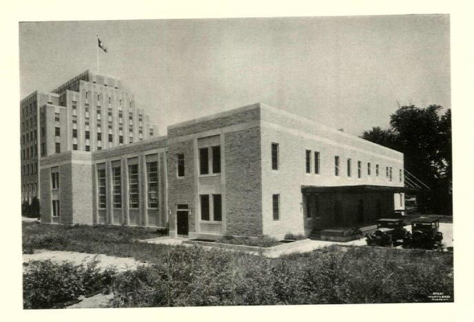
Above, a corner view from the rear, showing at the right the mailing platform. The only part of the building below grade is that under the rear end block, providing for boiler-room space and storage. Below, the workroom, which has a wood wainscot and wood block floor
