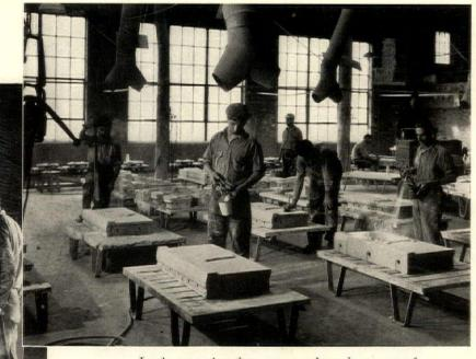
In the spraying department where, by means of compressed air, the exposed surfaces of the terra-cotta are covered with the ceramic mixture or "slip" which, in the firing, develops the desired color or glaze
