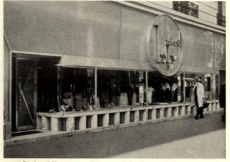
45 Boulevard Haussmann. The outer window frame, sill, base course, and basement "mullions" are of white marble with black veining. Basement grilles are dull silver in color. The broad expanse of gray semi-opaque glass above the show window is mottled, and not quite smooth. The circular sign has a silvery rim and letters, against an imitation mother-of-pearl background
