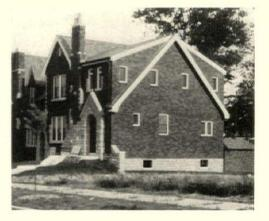
cottage. A high-pitch "cross-gable" was turned across the front of the house, giving it the appearance of running parallel to the street. The main roof being kept at a lower pitch, the fact was hidden from sight that the bulk of the house was arranged precisely as before. This ingenuity was cleverly manipulated in many Minneapolis examples but botched in other cities. The ubiquitous front chimney, badly placed for living with but easy to advertise, was also characteristic of this period.
