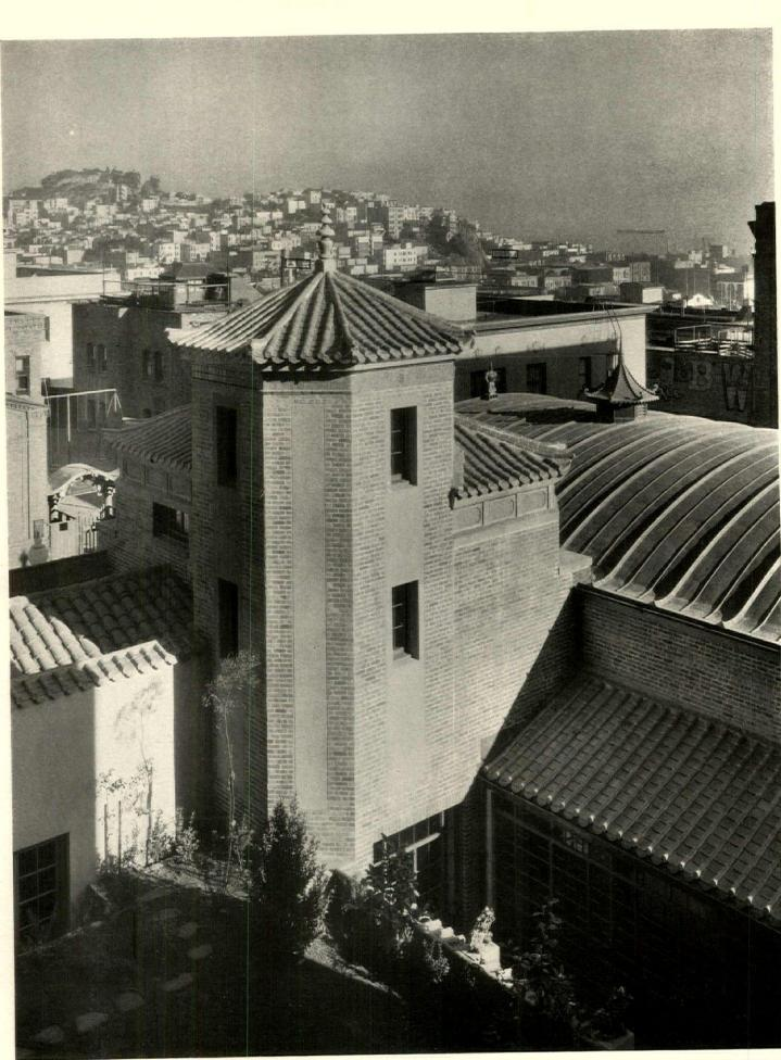
Detail of the east tower and roof composition. The nearer roofs are of handmade tile, the walls of brick and cast stone
