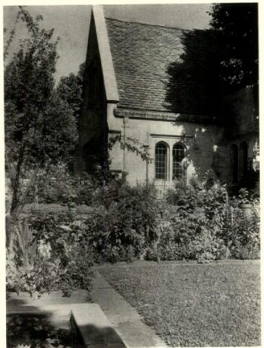
South end of the studio building and the low wall enclosing the garden. On the exterior Mr. Hopkins has used limestone four inches thick backed by cinder block. This limestone is in a mixture of channel-face and shot-sawn slabs, giving variety of texture and color
