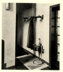
hanging of a coat by its tape through the use of the metal ring. Incidentally, the umbrella rack, it will be noticed, provides a small receptacle for the drip.
