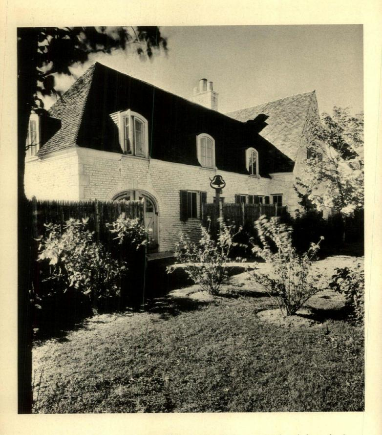
The service wing, with the garage space for a single car—there is a separate garage building elsewhere on the estate. The dormers are roofed with copper, the cheek walls being formed by the roof tile, carried across in corresponding courses. Garage doors are of natural oak. Chimney pots are natural clay color, darkening through use
