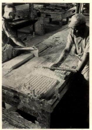
In the moulding shop. From the original models plaster moulds are here made. From these moulds an almost unlimited number of terra-cotta units can be manufactured, if desired
