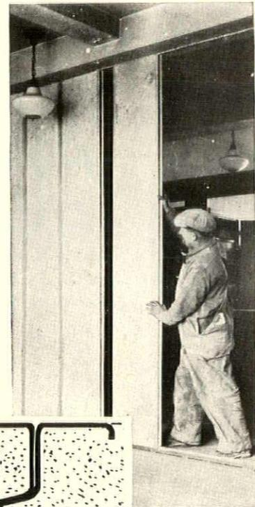
Showing how Plank, in meshing, form supporting steel I-beams 15" on centers.
