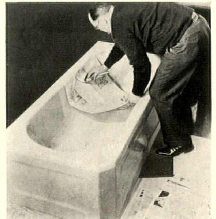
Applied with common paint brush. Hard covering that withstands all common abuses. Removed by soaking with water and peeling off. Kohler Company, Kohler, Wis.
