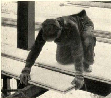
channel-like sections of galvanized copper-bearing steel, tongued and grooved like wood plank. Erected with random joints. Maximum spans, floors 4', roofs 6'. Structural Gypsum Corporation, Linden, N. J.
