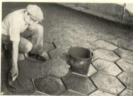
in patented brass strip, nailed to wood underflooring, in tile patterns, 1" thick. Information from National Terrazzo Assn., Portland Cement Assn., or from strip manufacturer, A. C. Horn Company, Long Island City, N. Y.
