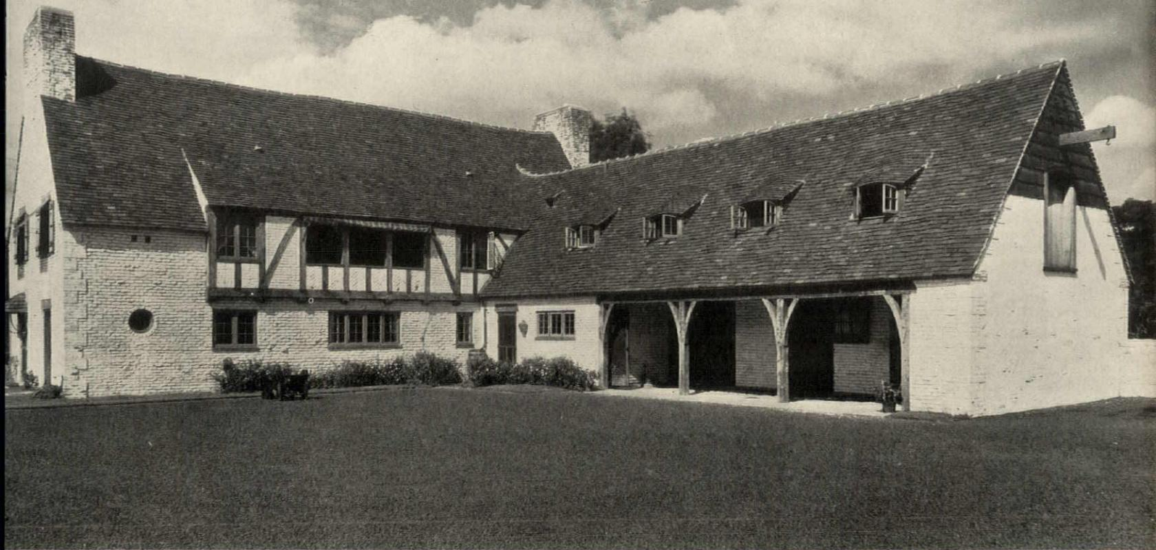
*The brick is whitewashed and, in parts, covered by stucco. The timbering, which is structural, is of oak, stained, whitewashed, and wire-brushed after a month or so*
