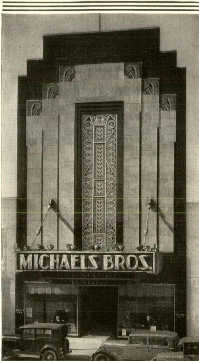
**MODERN:** The black is a lustrous glaze. The lighter color is polished aluminum. (*The metal is melted and applied at extreme heat directly upon the terra cotta.*) The parapet fern decoration is in sparkling polychrome colors... All an unusual bit of modern trade compelling architecture in Terra Cotta.
