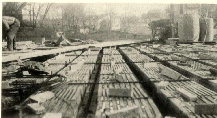
*The terra-cotta tile and reinforcing bars in place for the floor slab, ready to pour the concrete. On top of this a composition or tile floor may be laid, or wood flooring on loose sleepers*
